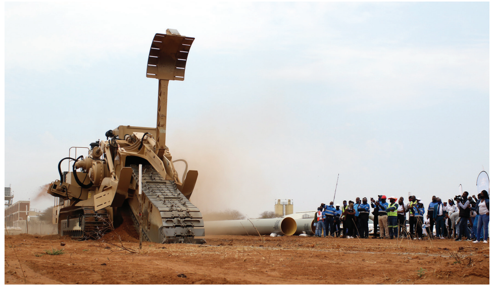
Ground breaking of Masama-Mmamashia pipeline
