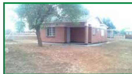
One of the staff houses at Tembwe Health centre renovated by Simbi Phiri
